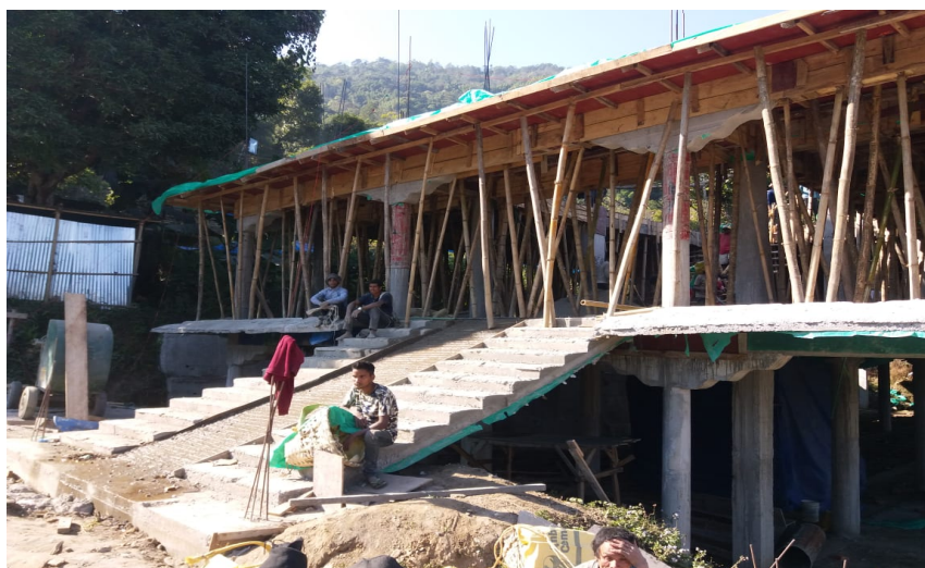
De school in aanbouw in Soreng in 2019
