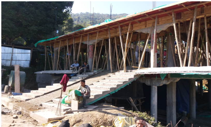
The school under construction in Soreng
